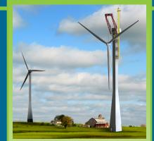
DOE Small Business Innovation Research (SBIR) support enabled Wind Tower Systems to develop the Space Frame tower, a new concept for wind turbine towers. Instead of a solid steel tube, the Space Frame tower consists of a highly optimized design of five custom-shaped legs and interlaced steel struts. With this design, Space Frame towers can support turbines at greater heights, yet weigh and cost less than traditional steel tube towers.
