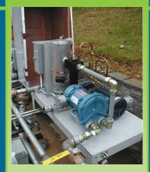
DOE Small Business Innovation Research (SBIR) support enabled CMS to develop a membrane vapor processor that recovers fuel vapors from gasoline refueling with 99 percent efficiency. This membrane system enables gasoline stations to surpass environmental regulations while reducing fuel losses.
