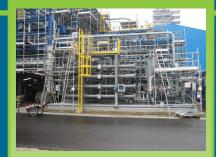
DOE EERE Small Business Innovation Research (SBIR) support enabled MTR to complete development of their VaporSep® process, which separates and recovers organic vapors from air and nitrogen. The process is now widely used to minimize monomer losses in polyolefin plant vent streams. For a world-scale polyolefin plant, a VaporSep® unit typically recovers about 2,000 to 200,000 tons/year of monomer, valued at \$1-10 million/ year.
