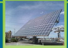
DOE Small Business Innovation Research (SBIR) support enabled Amonix to develop its 7700 system, which drastically reduces the requirement for costly solar cells by using Fresnel lenses to concentrate sunlight 500 times onto small, highly efficient photovoltaic cells. This reduces the cell area so that expensive solar cell materials can be replaced with inexpensive plastic lenses.
