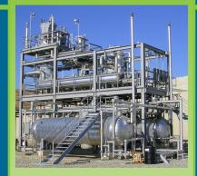
DOE Small Business Innovation Research (SBIR) support enabled TDA to develop and commercialize its direct oxidation process—a simple, catalyst-based system for removing sulfur from natural gas and petroleum—that was convenient and economical enough for smaller fuel processing plants to use.
